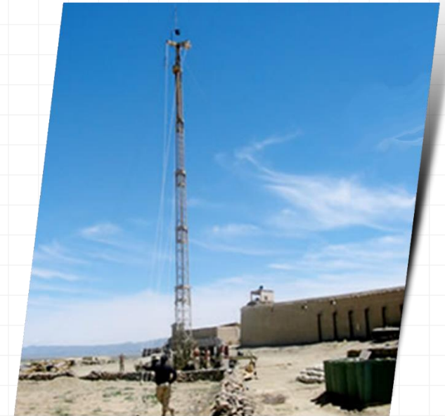
RAID towers provide persistent surveillance capability using infrared sensors elevated on a stationary platform.
